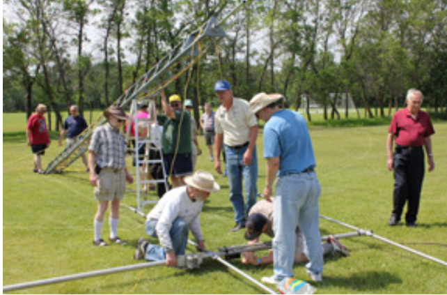
Like clockwork, well, sort of, the large crew was on hand to erect the HF beam. By 1300 hours local time VE4BB was on the air!
