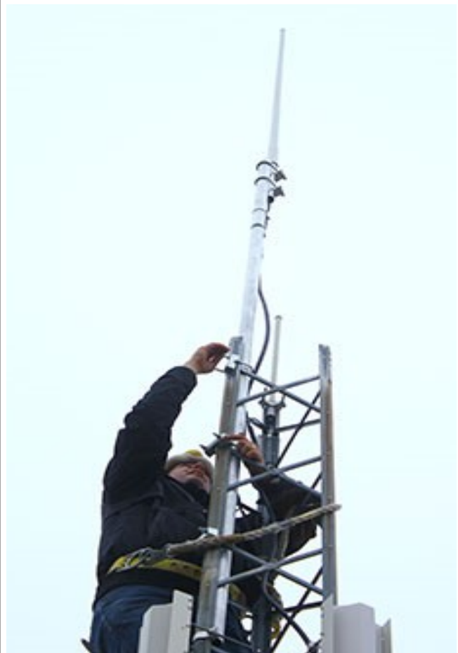
Garth VE4GWB securing the antenna mounting brackets
