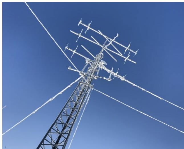
Looking up the tower, Alpha Delta 40-80 NVIS wire antenna, Alpha Delta 6-80 DX-CC wire antenna, 1.2 GHZ vertical, 5.8GHZ microwave data links, 2,3GHz vertical (data), Cushcraft MA5B mini beam for 10-12-15-17-20, Cushcraft A627013S beam 6m (horizontal), 2m/70cm (vertical). On a DMX medium 60' tower
